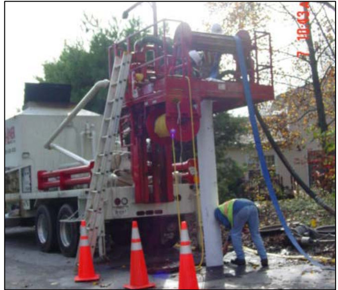
Truck mounted boiler for installing CIPP
